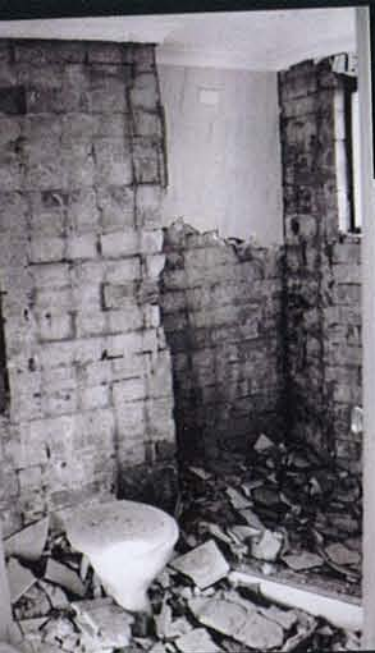
ABOVE: THE DEMOLITION OF MANY OF THE WALLS WAS POSSIBLE AS THE INTERNAL WALLS WERE NOT LOAD BEARING. BELOW: NARROW PIVOTING SHUTTERS CONNECT THE KITCHEN TO THE DINING AREA AND NORTHERN VIEW BEYOND. THE MAXALTO TABLE AND B&B ITALIA 'SOLO' CHAIRS, COVERED IN BURNT-ORANGE ULTRASUEDE, ARE FROM SPACE FURNITURE. THE MICHAEL SCHLIEPER PAINTING PICKS UP THE COLOUR ACCENTS. OPPOSITE PAGE: WINDOWSILLS WERE LOWERED TO SIT BELOW THE BACK HEIGHTS OF THE FLEXFORM 'GROUNDPIECE' SOFA. TO THE RIGHT, THE PIVOTING PANELS SHARE THE VIEWS WITH THE MASTER BEDROOM. THE ORIGINAL KITCHEN, BELOW RIGHT, WAS DOUBLED IN SIZE AND EXTRA WINDOWS WERE ADDED TO THE WESTERN WALL. BELOW LEFT, CABINETS ARE FINISHED IN SATIN POLYURETHANE WITH A STAINLESS STEEL ISLAND AND SMALL EAT-IN AREA.
