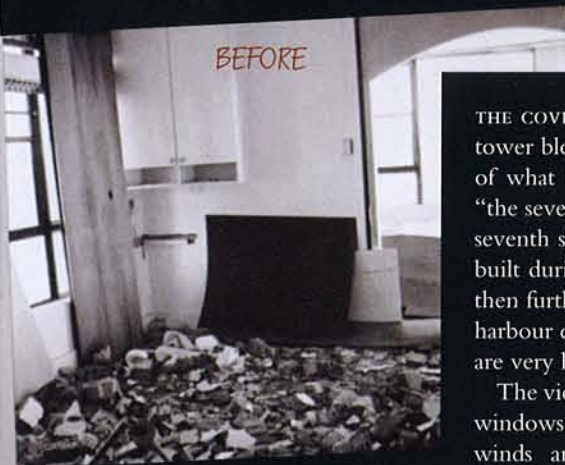
ABOVE: THE DEMOLITION OF MANY OF THE WALLS WAS POSSIBLE AS THE INTERNAL WALLS WERE NOT LOAD BEARING. BELOW: NARROW PIVOTING SHUTTERS CONNECT THE KITCHEN TO THE DINING AREA AND NORTHERN VIEW BEYOND. THE MAXALTO TABLE AND B&B ITALIA 'SOLO' CHAIRS, COVERED IN BURNT-ORANGE ULTRASUEDE, ARE FROM SPACE FURNITURE. THE MICHAEL SCHLIEPER PAINTING PICKS UP THE COLOUR ACCENTS. OPPOSITE PAGE: WINDOWSILLS WERE LOWERED TO SIT BELOW THE BACK HEIGHTS OF THE FLEXFORM 'GROUNDPIECE' SOFA. TO THE RIGHT, THE PIVOTING PANELS SHARE THE VIEWS WITH THE MASTER BEDROOM. THE ORIGINAL KITCHEN, BELOW RIGHT, WAS DOUBLED IN SIZE AND EXTRA WINDOWS WERE ADDED TO THE WESTERN WALL. BELOW LEFT, CABINETS ARE FINISHED IN SATIN POLYURETHANE WITH A STAINLESS STEEL ISLAND AND SMALL EAT-IN AREA.
